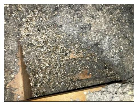
PHOTOGRAPH #27: Vermiculite - Attic (<1% Actinolite)
