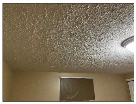
PHOTOGRAPH #7: Ceiling Texture - Basement Bedroom (None Detected)
