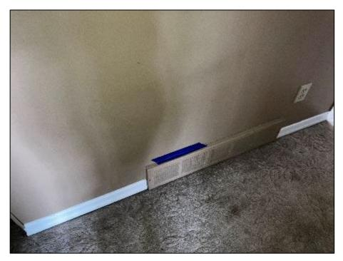
PHOTOGRAPH #28: Paint - Level 1 Hallway Brown (160 ppm Lead)
