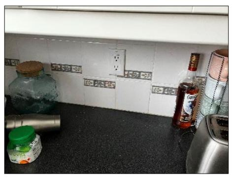
PHOTOGRAPH #26: Thinset and Adhesive - Level 1 Kitchen (None Detected)
