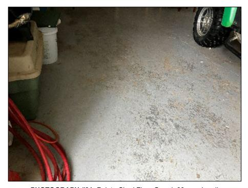
PHOTOGRAPH #31: Paint - Shed Floor Grey (<80 ppm Lead)
