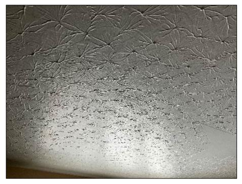
PHOTOGRAPH #5: Ceiling Texture - Level 1 Living Room Lace (None Detected)
