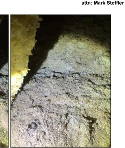
2.4 Item 1(Picture) Attic Insulation - signs of tunneling 2.4 Item 2(Picture) Attic Insulation - signs of tunneling from rodents
